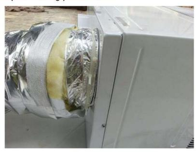
(The thick cotton tube in the transparent plastic bag is the cold air connection tube.)
