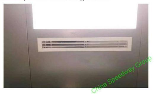
7. If the temperature in the elevator shaft is relatively high, it can adversely affect the cooling efficiency and lifespan of the air conditioner. In this case, connect the return air duct. Simply attach the insulated return air duct directly to the return air opening using insulation foam. (The return air opening must lead directly into the elevator cabin interior).
