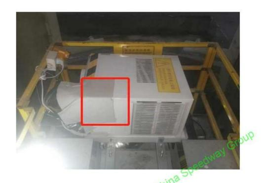
4. Place the air conditioner steadily on the supporting base on the cabin top. Position two angle irons parallel to each other as shown in the diagram. Secure the unit's chassis using four "Z-shaped brackets," align the holes, and fasten the condensate water tray using screws and other provided hardware. After fixing the bracket, check that both the chassis and the main unit are level and securely fastened.
