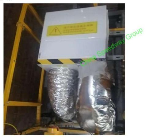
3. Apply a layer of insulation foam (300mm width x 600mm length) from the front top edge of the cold air outlet down to the metal reinforcement rib. Position it vertically at a 90-degree angle. This prevents water droplet condensation around the cold air outlet during continuous cooling operation over several days.
